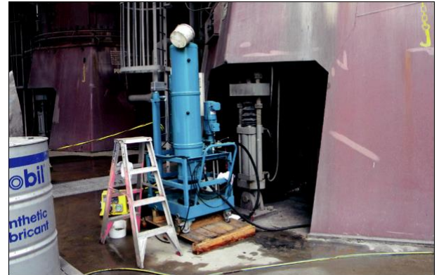
Millmerran Power Station, coal-fired power plant, Australia, with the CJC™ Filter Separator PTU3 27/108 P installed
