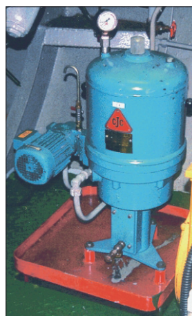
PTU2 27/27 P for gas oil separation
