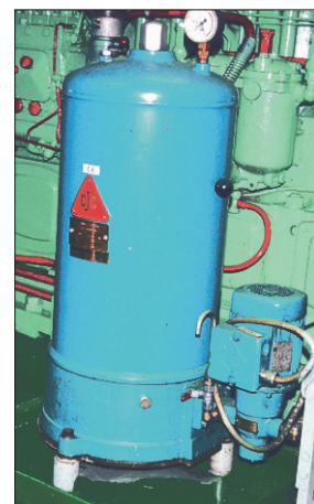
HDU 27/54 P for lube oil treatment
