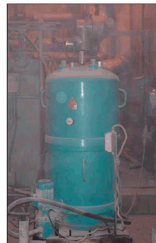
CJC™ Fine Filter HDU 427/108 installed
