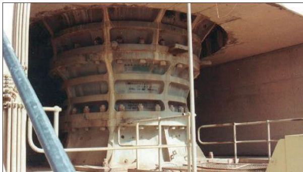
BHP Billiton, Minera Escondida, Primary Crusher
