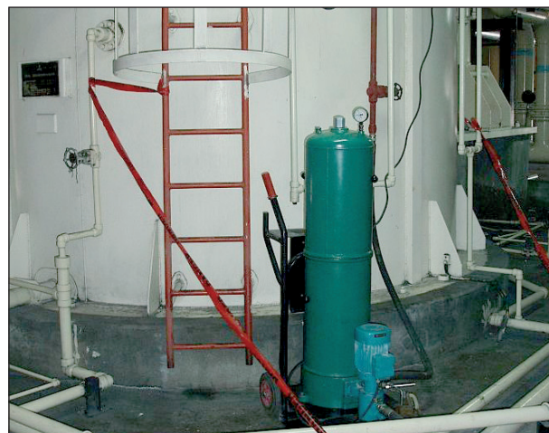
The CJC™ Fine Filter HDU 27/108 installed at one of the Steam Turbine Tanks at AES Masinloc, Luzon
