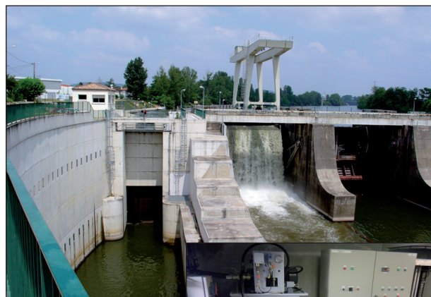
EDF Hydroelectric Dam France
