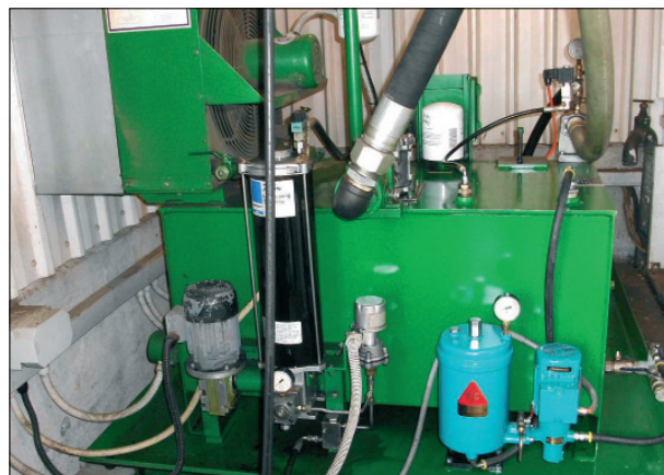
The Hydraulic Power Pack at Taranaki Pine, New Zealand with the CJC™ Fine Filter HDU 15/25 PV installed
