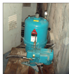
CJC™ PTU2 27/27 PV installed at the hydraulic system of the vertical raw mill, #4
