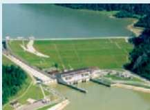
Water Power Plants Group Niedzica S.A, Poland
