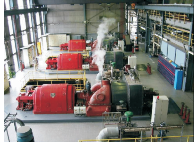
Steam Turbines at AVR Rotterdam.
