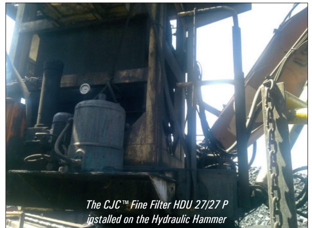
The Hydraulic Hammer at Exxaro Grootegeluk Coal Mine
