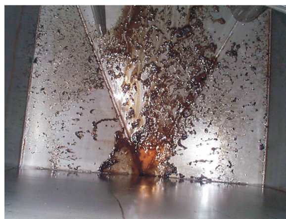
Fig. 1: Hydraulic oil tank on offshore-application
